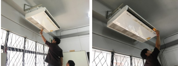
Figure 6. Measuring of temperature and relative humidity of return and supply air.
