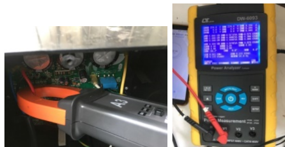
Figure 8. Electric power measurement and recording.
