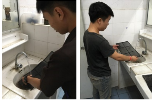
Figure 10. Air filter cleaning.
